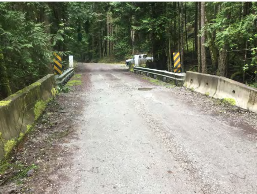
Approach from Left Bank when facing downstream
