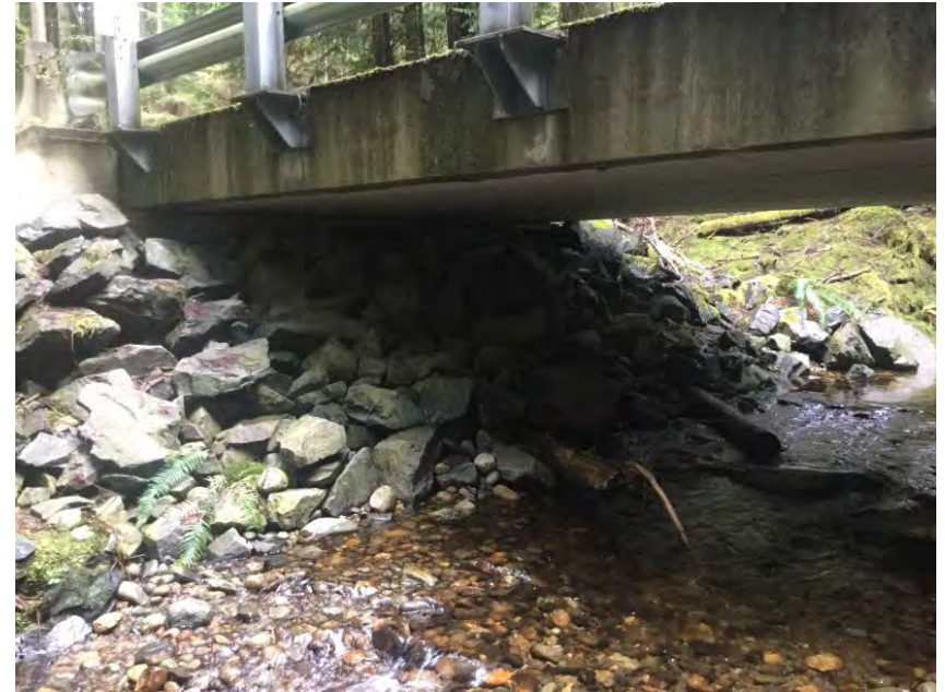
Right Bank Abutment when facing downstream
