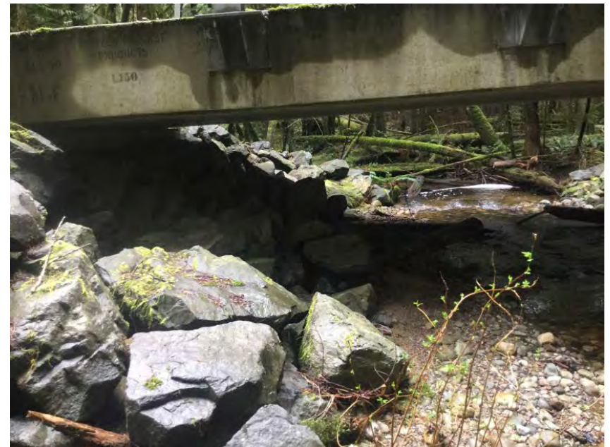
Left Bank Abutment when facing downstream
