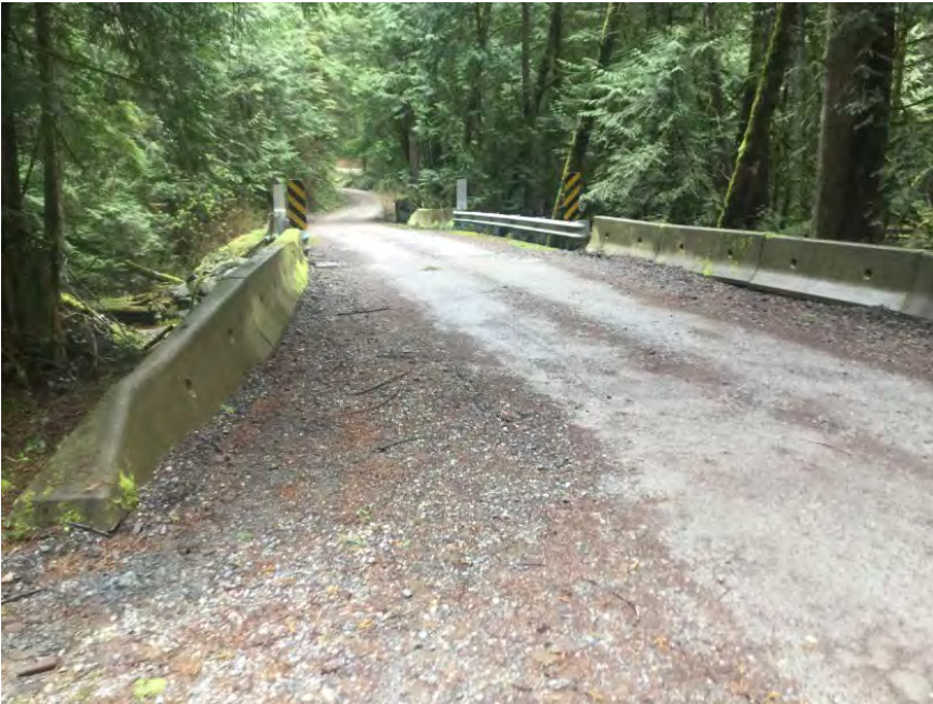
Approach from Right Bank when facing downstream
